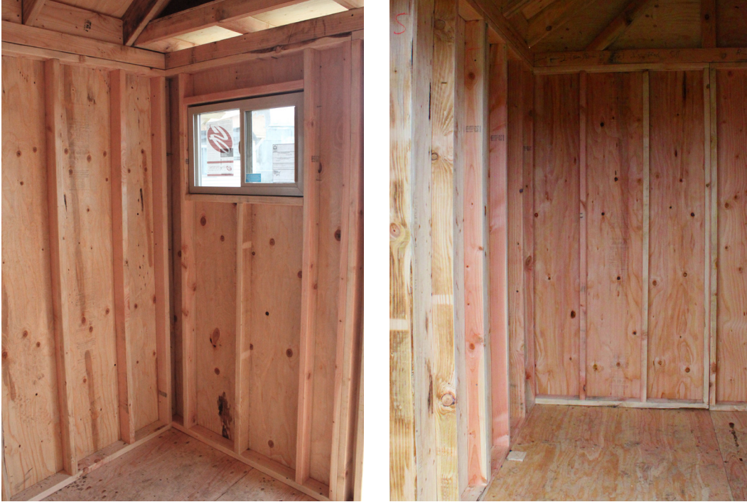
Figure 36: VIEW OF BUNGALOW INTERIOR STRUCTURE
